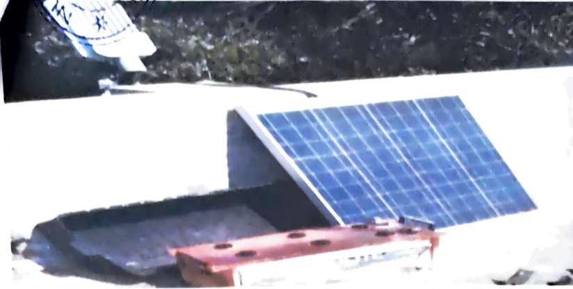
Solar Units Photo
